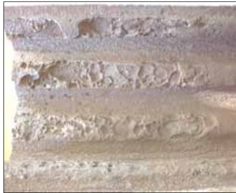
Radiant Coil Hot Spot Damage
